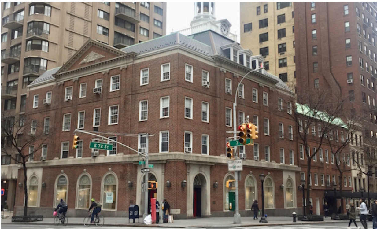
1251 Third Ave., the new location for a Morton Williams grocery
